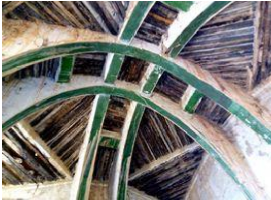
Fig. 8: Roof truss. Source, Author's archive. November 2017
