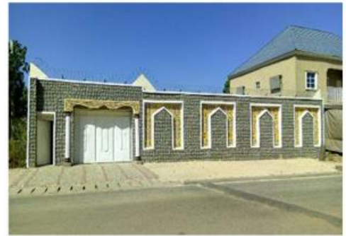
Fig. 6: Stone wall finishing Source: Author's field photos. Nov 2017
