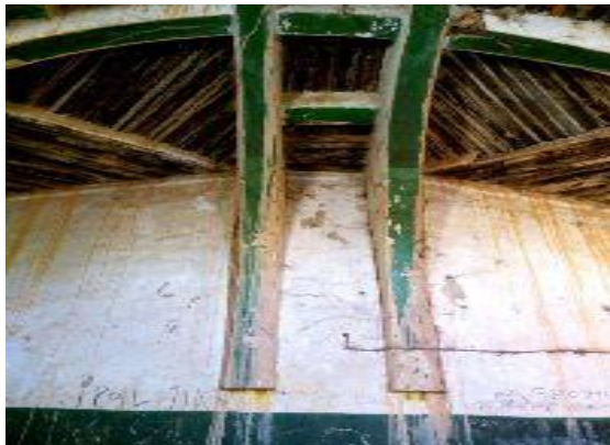
Fig. 9: Roof beams supported by corbels in walls Source, Author's archive. November 2017
