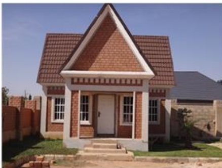
Fig.3: House constructed using CEB technology in Katsina. Source: Author's Archive. Nov 2017.
